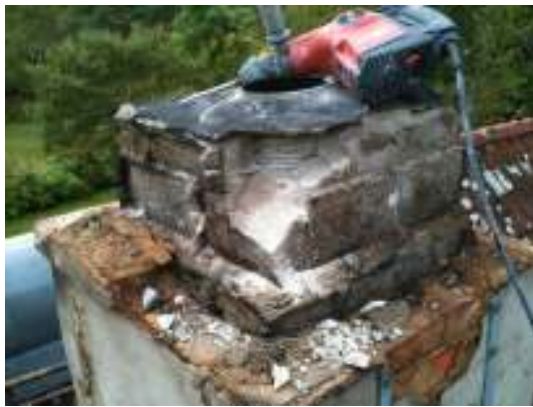
Fig. 2. "Betongplugg" i skorstenspipan.
