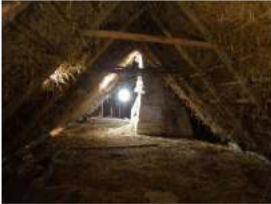
Illaren innan nedmontering.
